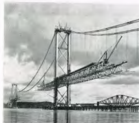
More than two tons of 'Terylene' have been used in the manufacture of the largest synthetic fibre nets ever made in Britain. Now installed beneath the road section of the Firth of Forth road bridge, the nets have a total area of 100,000 sq. ft. The roadway section is 180 ft. above the water and is being built out from either side of the two main towers. Four separate nets, slung on frames 35 ft. below the roadway, cover the areas where some 70 men are working and are moved as construction proceeds.
